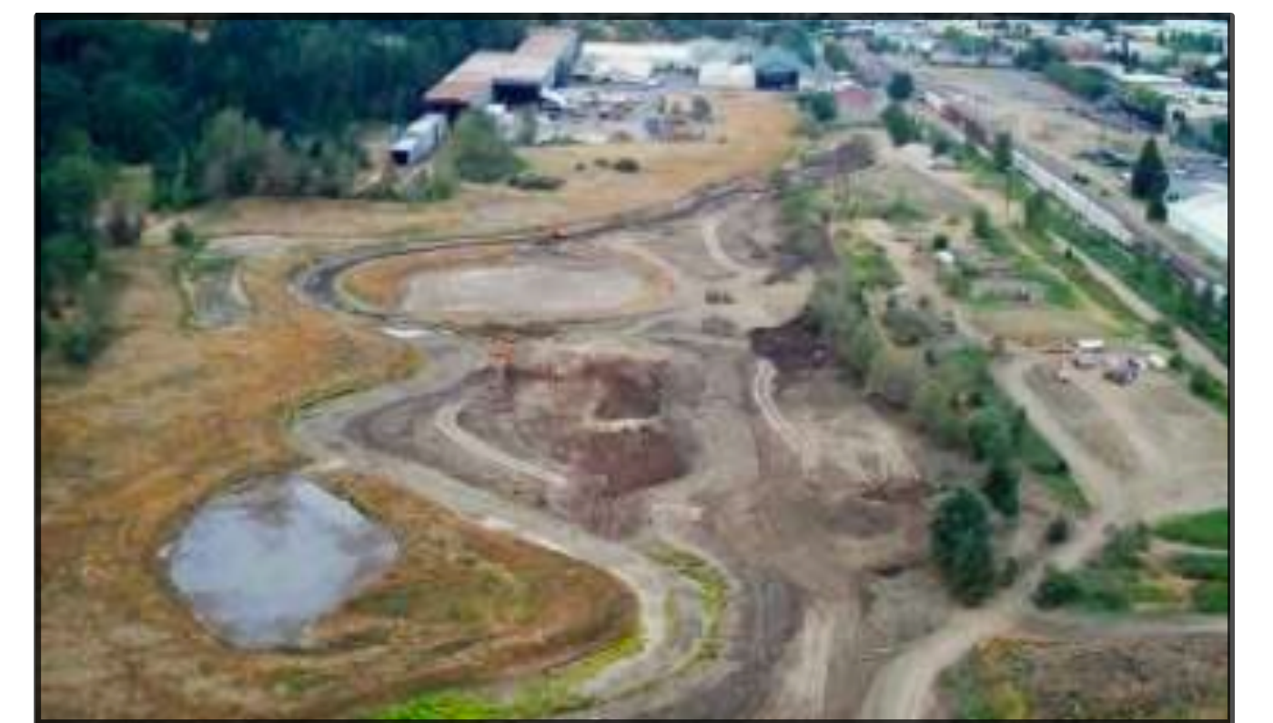
Springfield is working to redevelop former mill sites.
