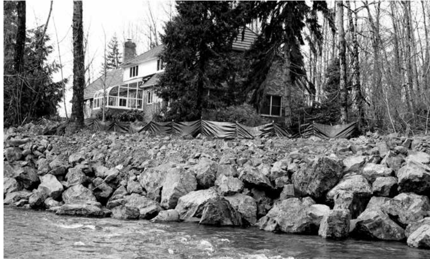
Riprap destroys habitat, creates downstream erosion and protects a permitted house where it doesn't belong on the McKenzie River
